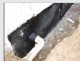
COUNTER FLASHING TO TORCHED MEMBRANES
